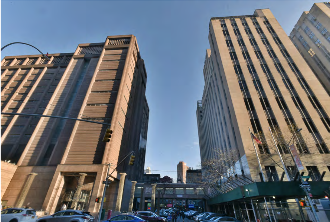
Under the city's plan, the north and south towers of the Manhattan Detention Center (24 White Street, right, and 125 White Street) would be demolished and replaced by a jail as tall as 50 stories. Photo: Carl Glassman/Tribeca Trib
